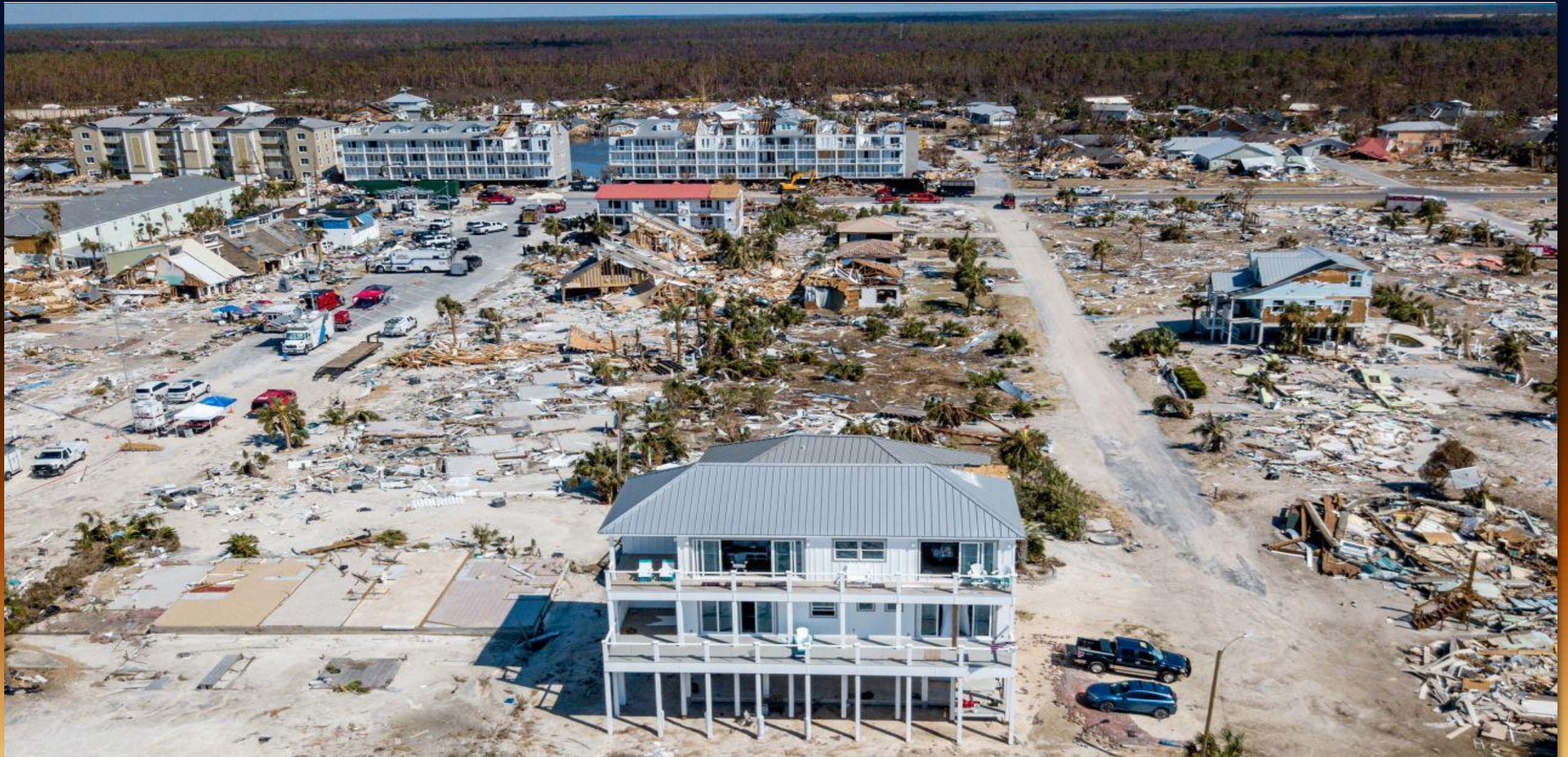
Home named Sand Palace (foreground) with surrounding structures demolished by Hurricane Michael in 2018. Image credit: Johnny Milano/The New York Times/Redux
