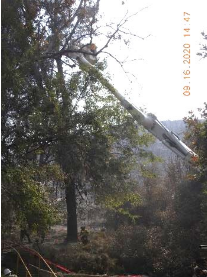
Figure 4: SCE field personnel preparing to lower the subject conductor.
