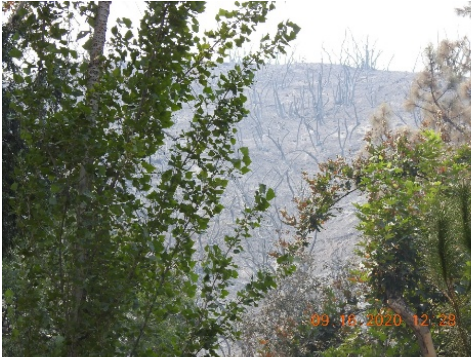
Figure 3: View from outside the USFS restricted area. The subject conductors are no longer supported by the H-frames and are lying across the ground.
