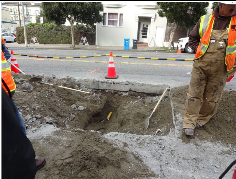
Figure 2. Photo of abandoned service tee location looking northwest towards 3976
