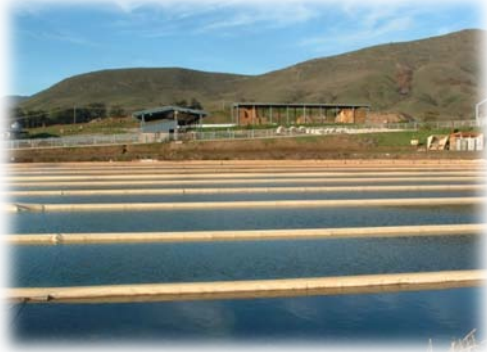
Animal waste from dairies and other livestock is often disposed of in man-made lagoons. Within these lagoons the waste undergoes a biological process that converts the waste into methane. This methane is often allowed to vent to the atmosphere.
