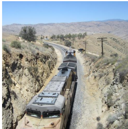
Westbound freight train exiting Tunnel #3 in Tehachapi Pass (Local Safety Hazard Site No.16)
