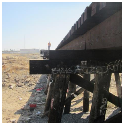
Railroad Bridge Evaluation Project – inspecting a wooden trestle in October 2013
