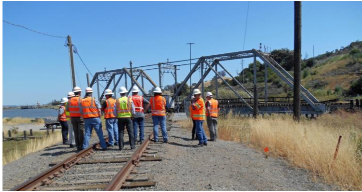
The group traveled by hi-rail over the Haystack Bridge which was then turned to allow passage of boat traffic on the Petaluma River. This bridge will be replaced.
