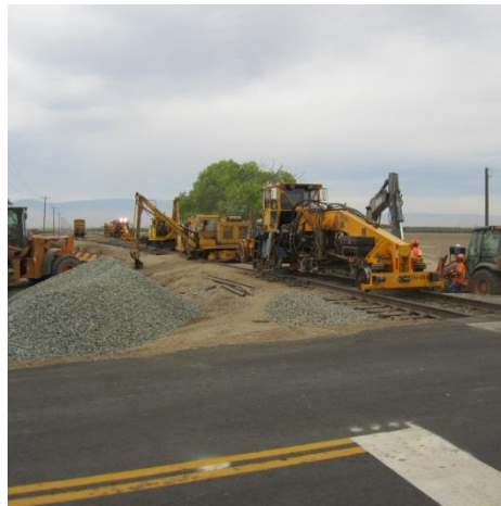
Rehabilitation along the Sunset Subdivision, southwest of Bakersfield, in preparation for crude oil train traffic.
