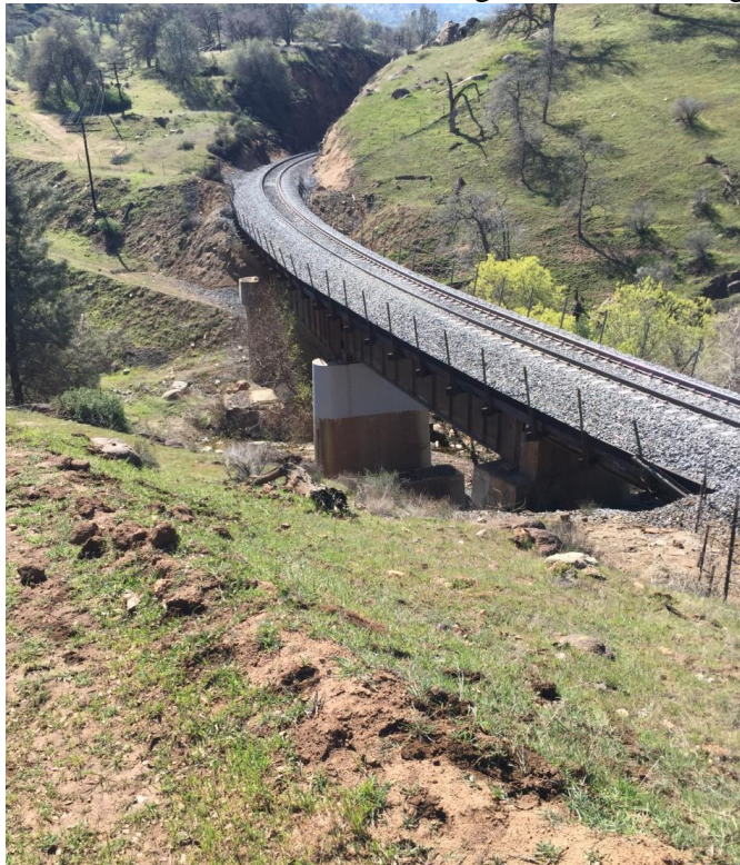
Both curves and grade territory are factors taken into consideration when choosing which bridges to examine. Bridge in the Tehachapi Pass area was chosen for observation as it features both.
