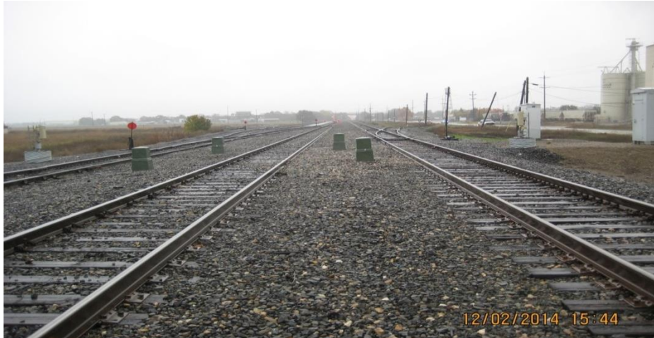
View looking South of Industrial Road, stationary green equipment boxes in walkway within 8' 6" of track center could strike an employee riding the side of equipment (Freight cars can extend 3 ft. beyond the rail)
