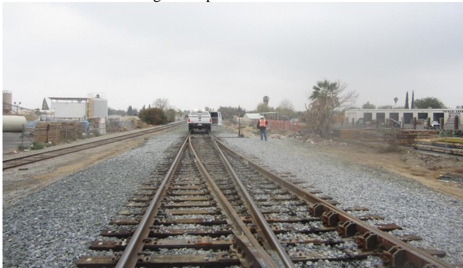
CPUC Railroad safety inspector-CORT member inspecting a switch
