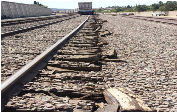
Track damage at Esperanza derailment site
