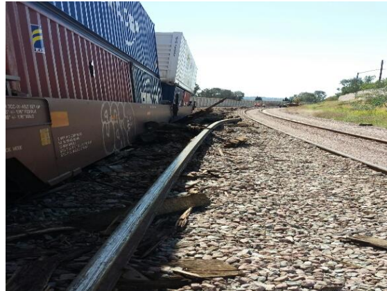
Track damage at Esperanza derailment site
