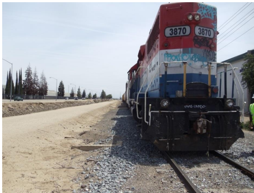
Remnants of an old concrete structure to the left of the locomotive are a tripping hazard and could lead to injury of crew members getting on or off the locomotive.
