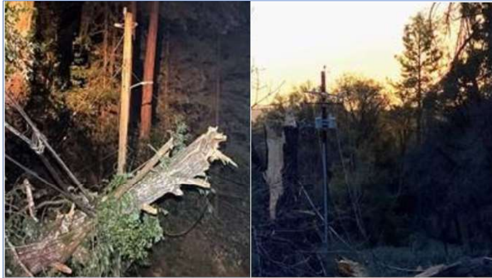
Figure 2-11 January 2021 Windstorm Damage
