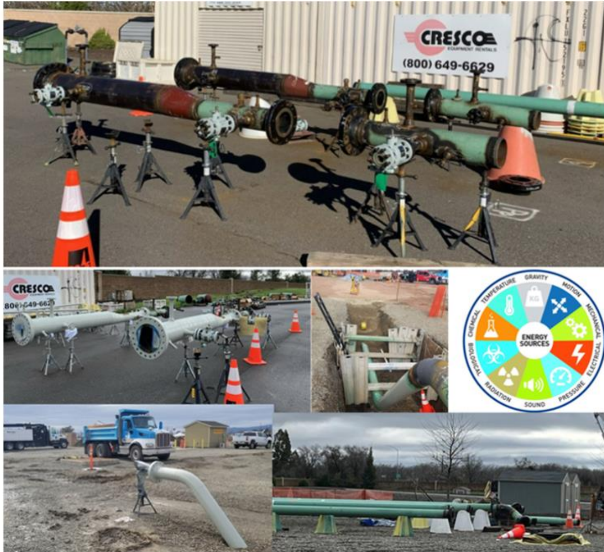
Figure 23: New Construction of the new Training Pigging Loop
