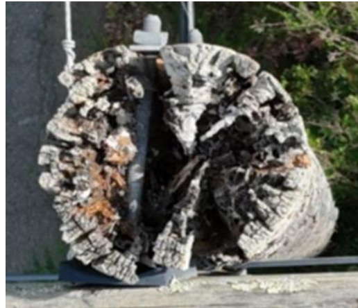
Figure 10: Examples of Defects Detectable by Aerial Inspection 19
