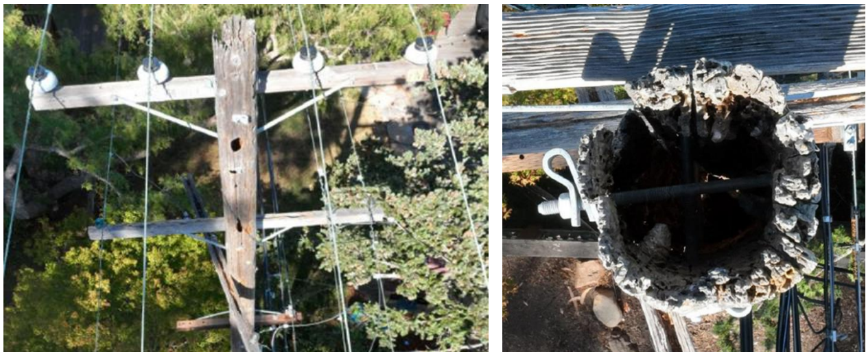
Figure 17: Aerial Cancellation of Ground Finding B Tag and Upgraded to an A Tag
