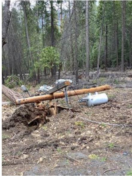
**Figure 16: Vegetation-Caused Damage in Madera County – Tree Fell Breaking Pole and Conductor**
