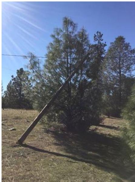
**Figure 19: Vegetation-Caused Damage in Mariposa County – Fallen Tree Broke Top Half of Pole Off**
