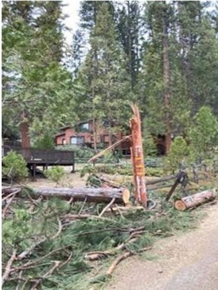
**Figure 15: Vegetation-Caused Damage in Mariposa County – Tree Took Down Lines and Broke Pole**
