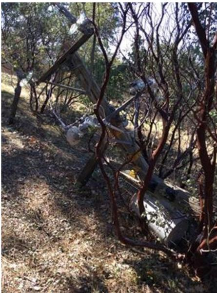
**Figure 18: Vegetation-Caused Damage in Mariposa County – Tree Fell Through Service Breaking Pole**
