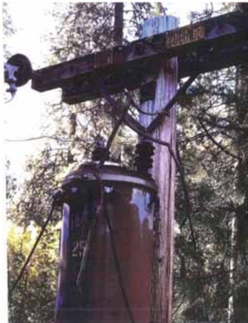
*Figure 2-In Nevada City, Nevada County, a tree branch on PG&E conductor. Brunswick 1105 circuit. Address: 10901 MILL SPRINGS DR, Nevada City*
