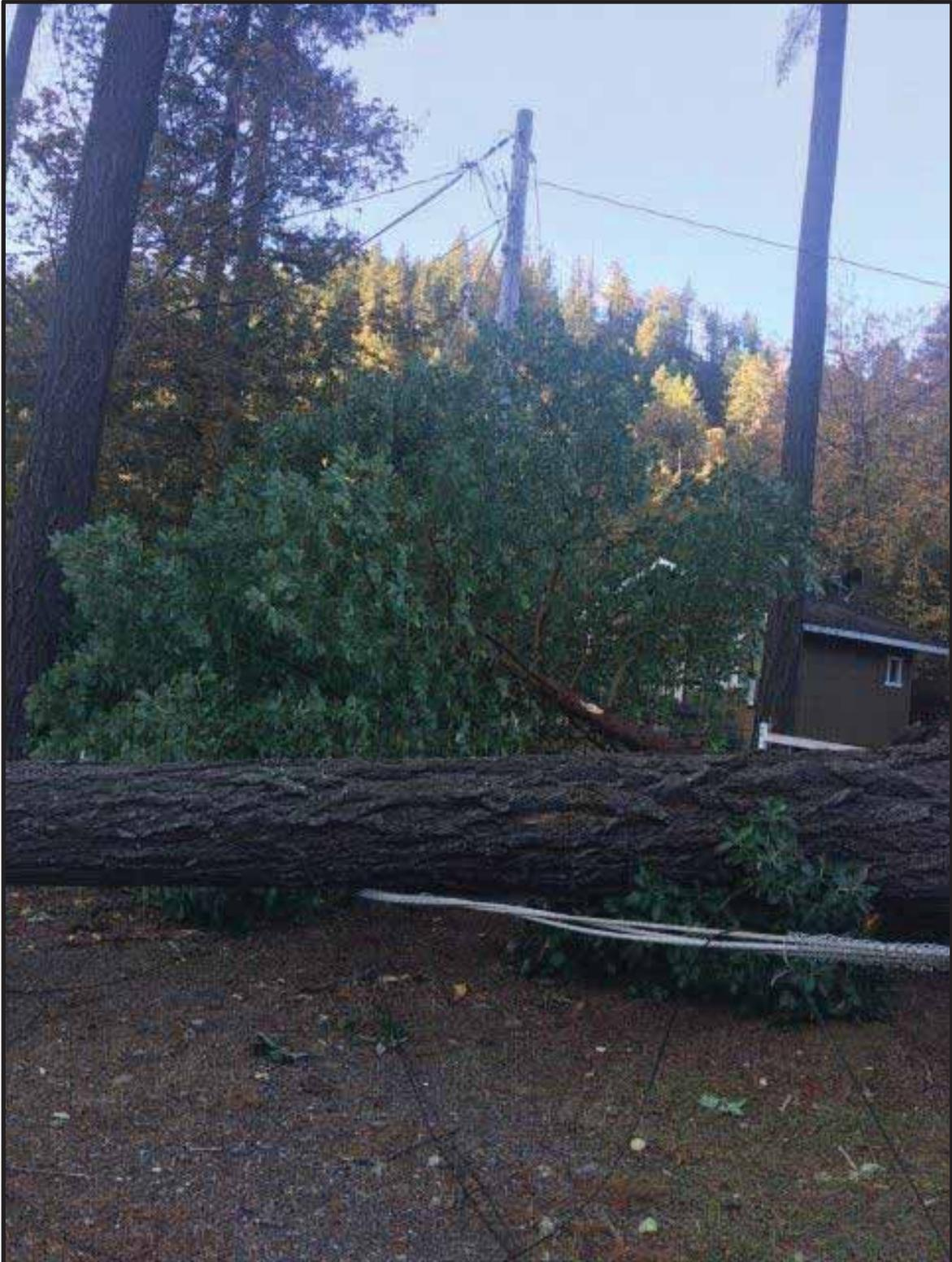
*Figure 3: Tree fell onto conductors; Unincorporated area of Santa Cruz County*
