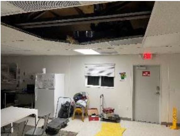
Figure 22. Navigation Center food preparation area.
