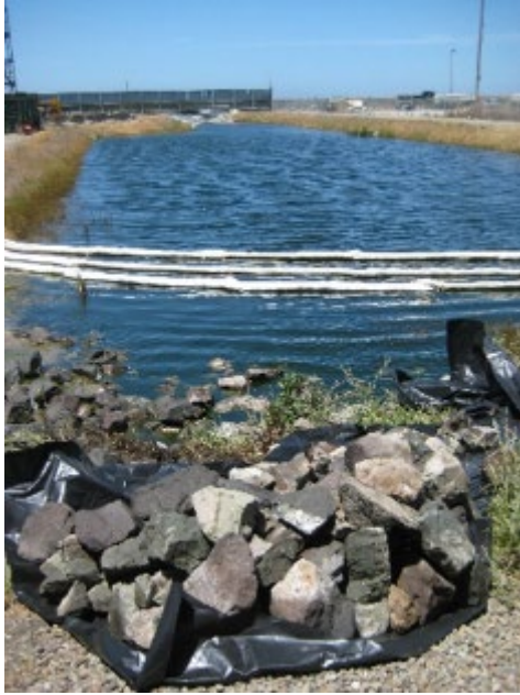
Figure 18. The water retention pond and the oil retention booms in service.
