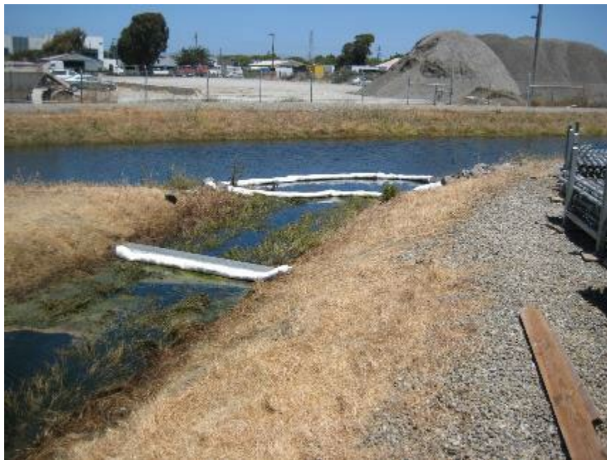
Figure 17. The storm water runoff canal and oil absorbing socks in use.
