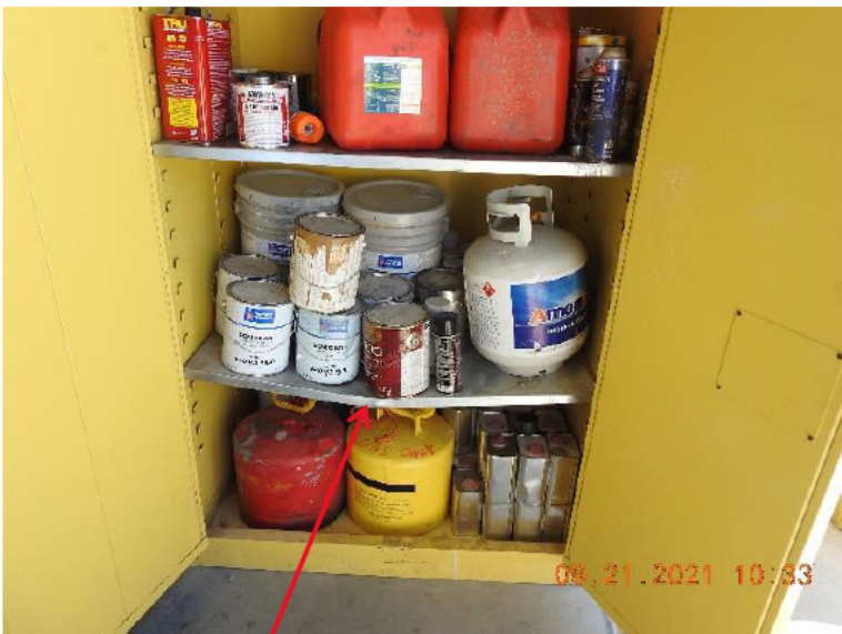
The middle shelf in the cabinet is sagging under the weight of the containers.
