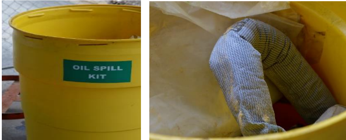
Figure 4: Oil Spill Kit had deteriorated stuff inside due to rainwater entering the drum
