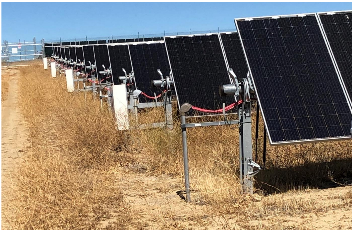
Figure 5: Dead vegetation that has grown to the bottoms of the solar panels
