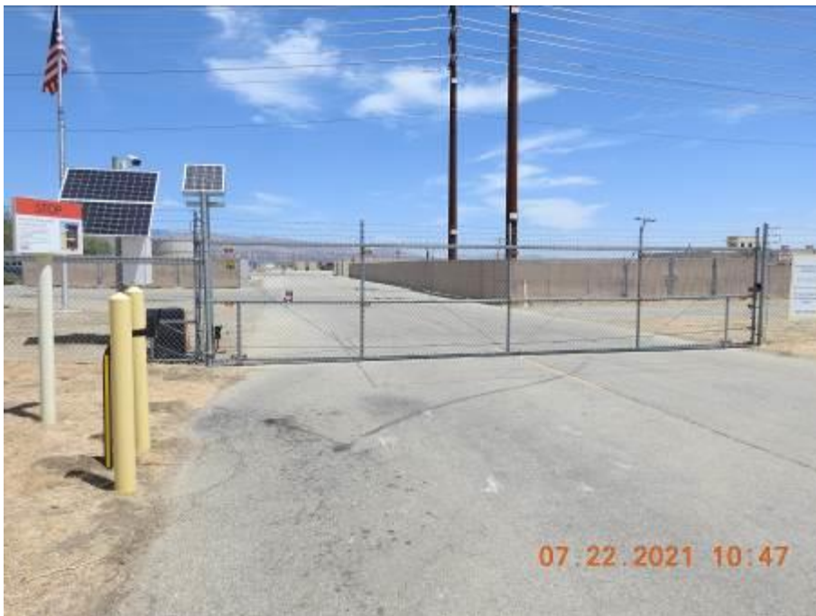
Missing NFPA Placard on the main gate.
