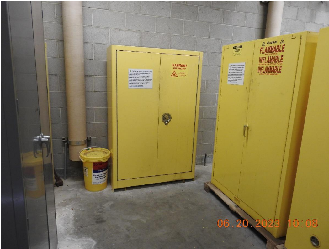
Figure 5: Missing NFPA Fire diamonds on the flammable storage cabinets
