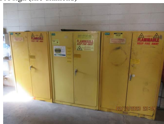
Figure 7 & 8: NFPA Fire diamonds missing on the flammable storage cabinets
