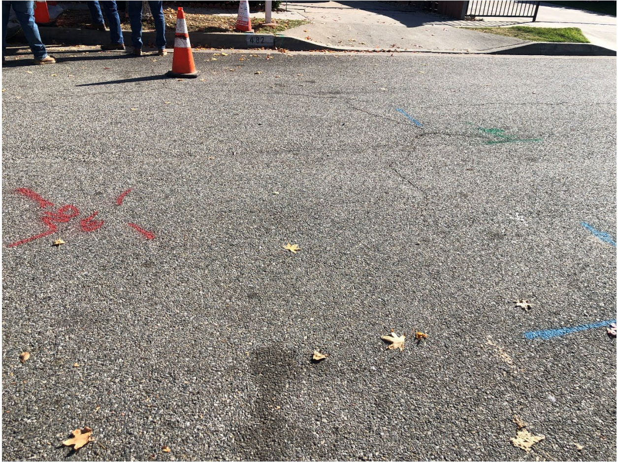
Photo 3. West View 2 (other pre-existing underground utilities' markings)
