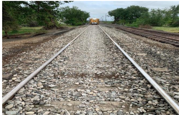
Bridge removed, main track reopened
