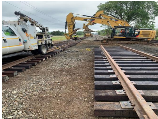
Last track panel placed on controlled siding
