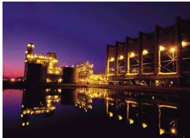
542 MW Sutter Energy Center
