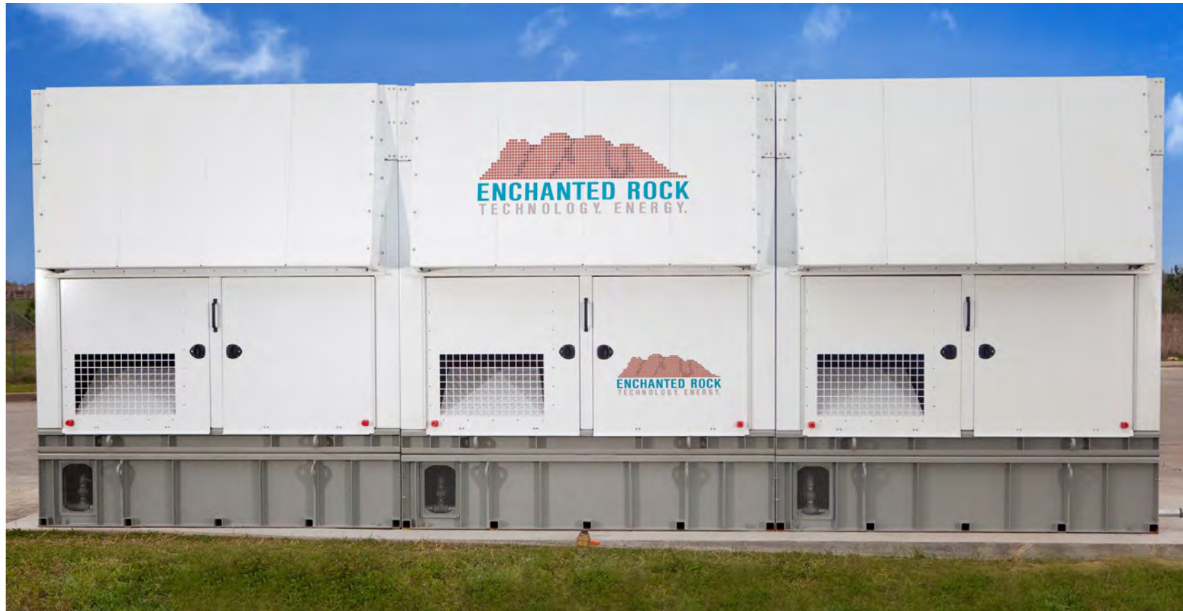
Three 448kW Genset Units
